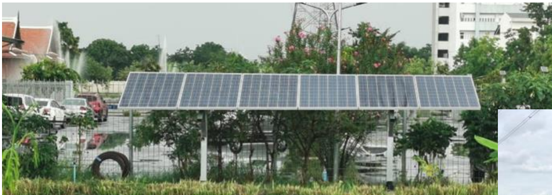
Polycrystalline silicon 1.56 kW
